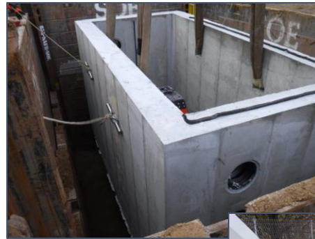
Vault Installation
